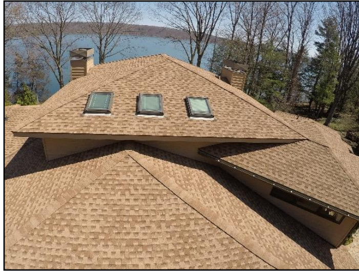
7. Asphalt shingles
