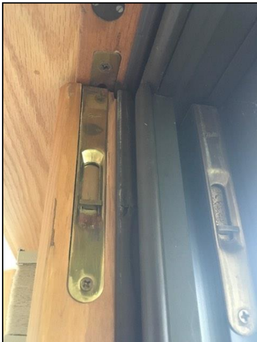
30. Does not latch properly
