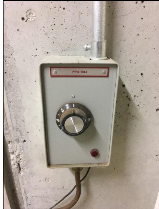
15. Footer drain heater
