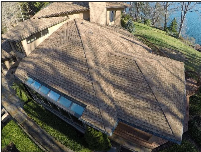
1. Asphalt shingles
