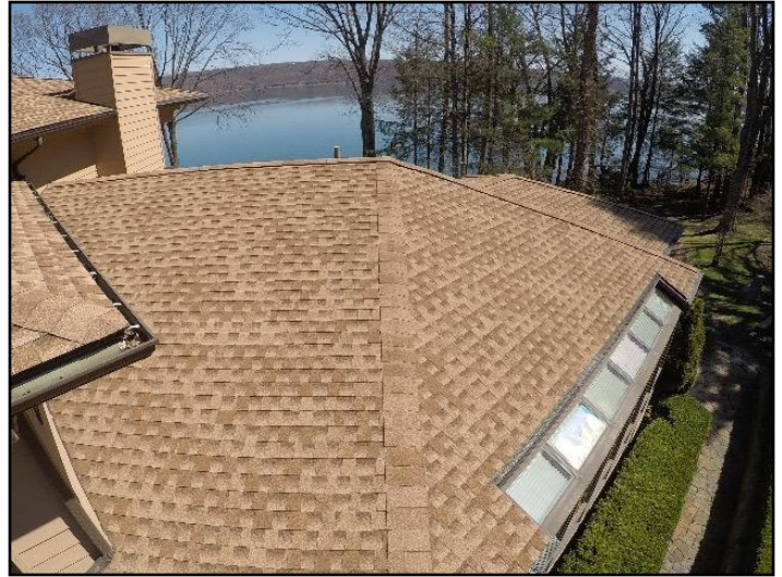
4. Asphalt shingles
