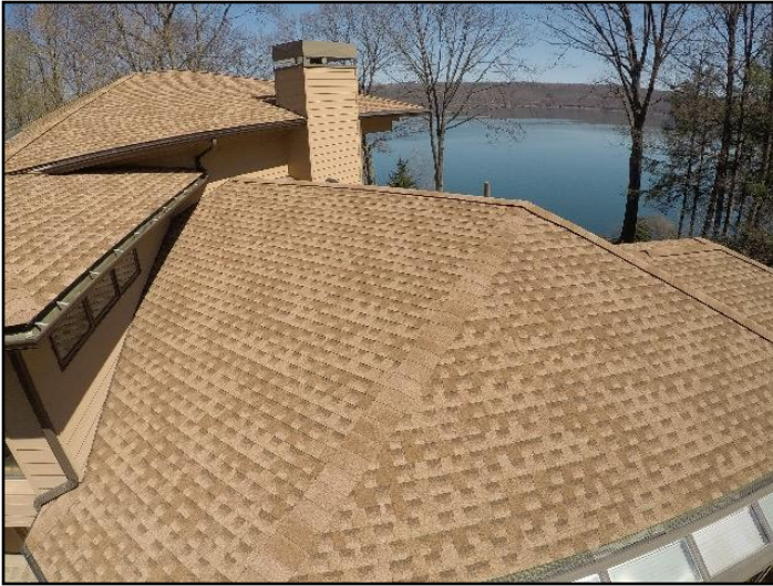
3. Asphalt shingles
