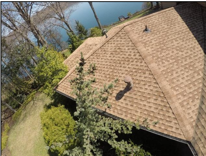
5. Asphalt shingles
