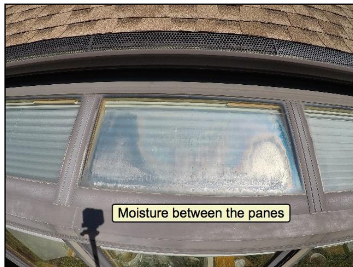
26. Lost seal on double or triple glazing
